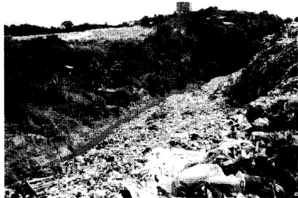
**Fig. 5.** Active and abandoned landfills: steep, uncovered slope (Source : Shoichi Hayami, 2007).
